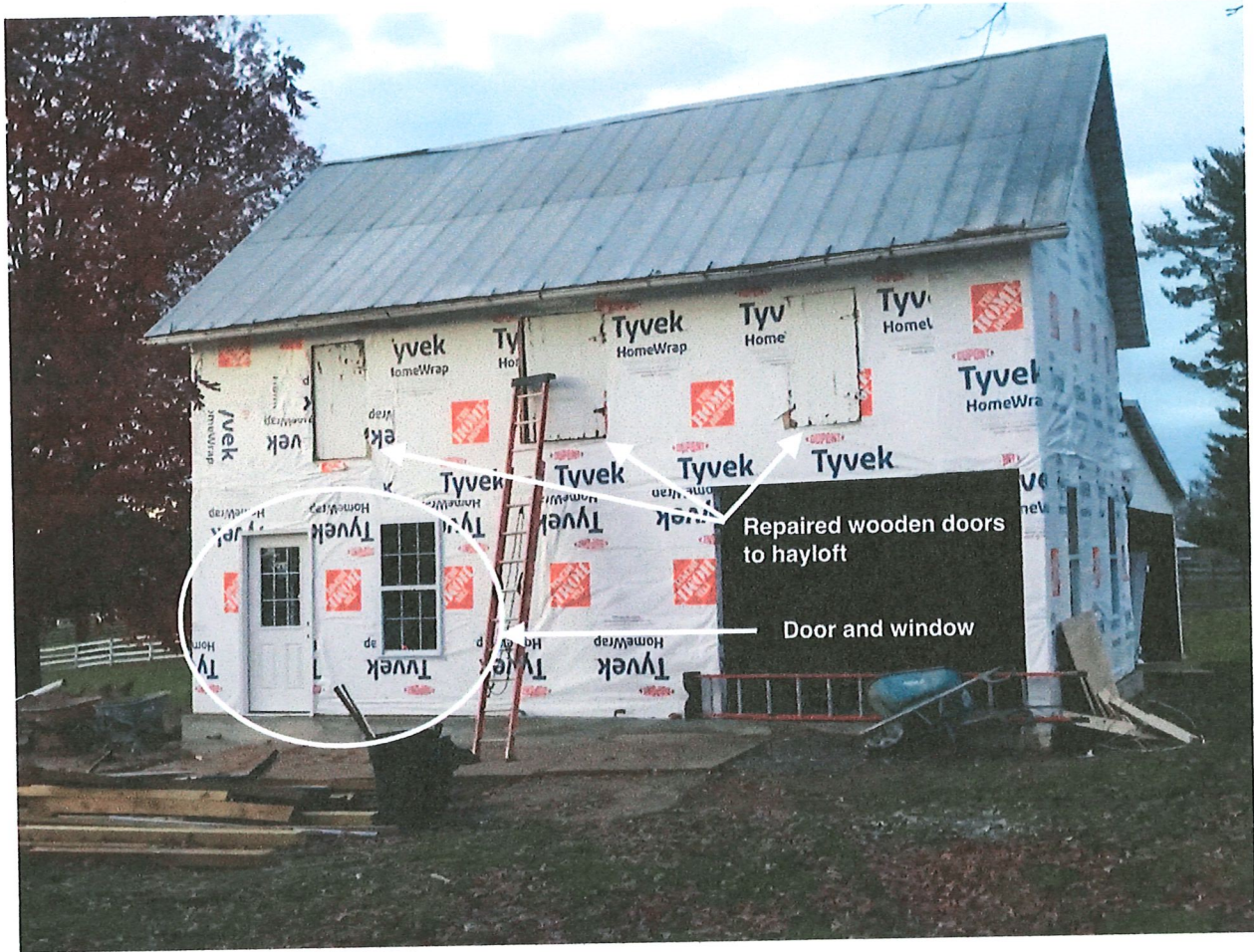
Front view (South side)
