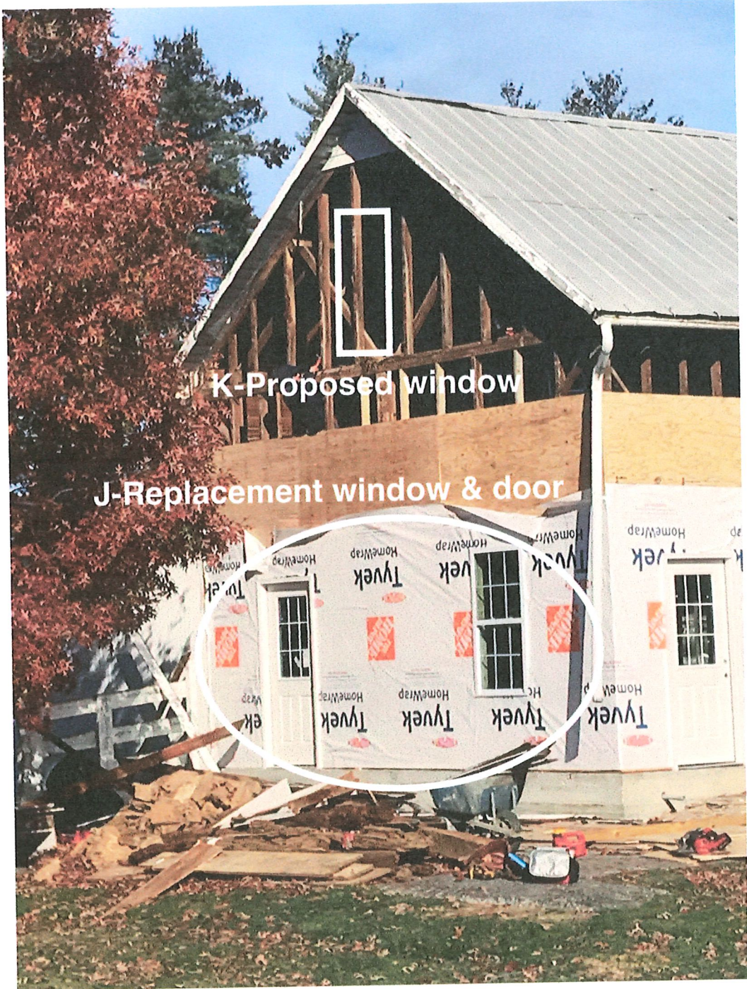
West Side (door & 2 windows)
