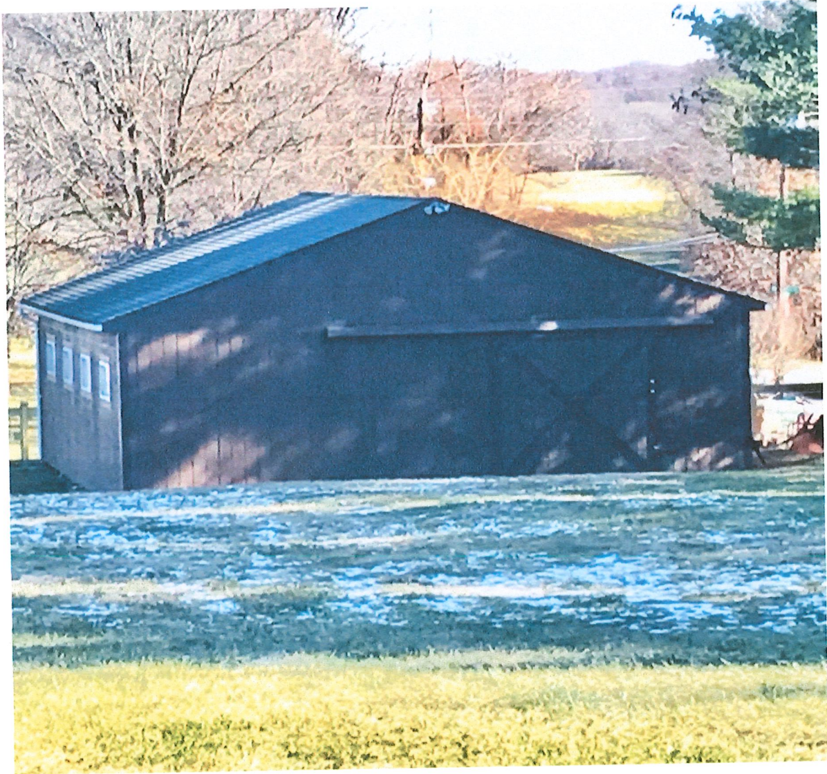
Another local example of a local instantiation of large wooden door (Griffith Road barn) on an overhead track.
