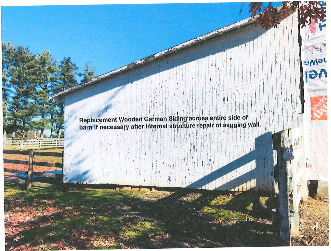
West rear side (not visible from Brink Road)
