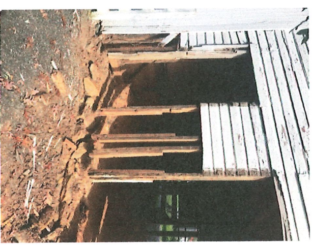
Attempts to reattach bottom board with nails or screws resulted in siding disintegrating with each turn of the screwdriver or pounding of the hammer
