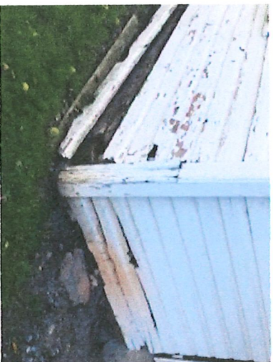
Attempts to reattach bottom board with nails or screws resulted in siding disintegrating with each turn of the screwdriver or pounding of the hammer
